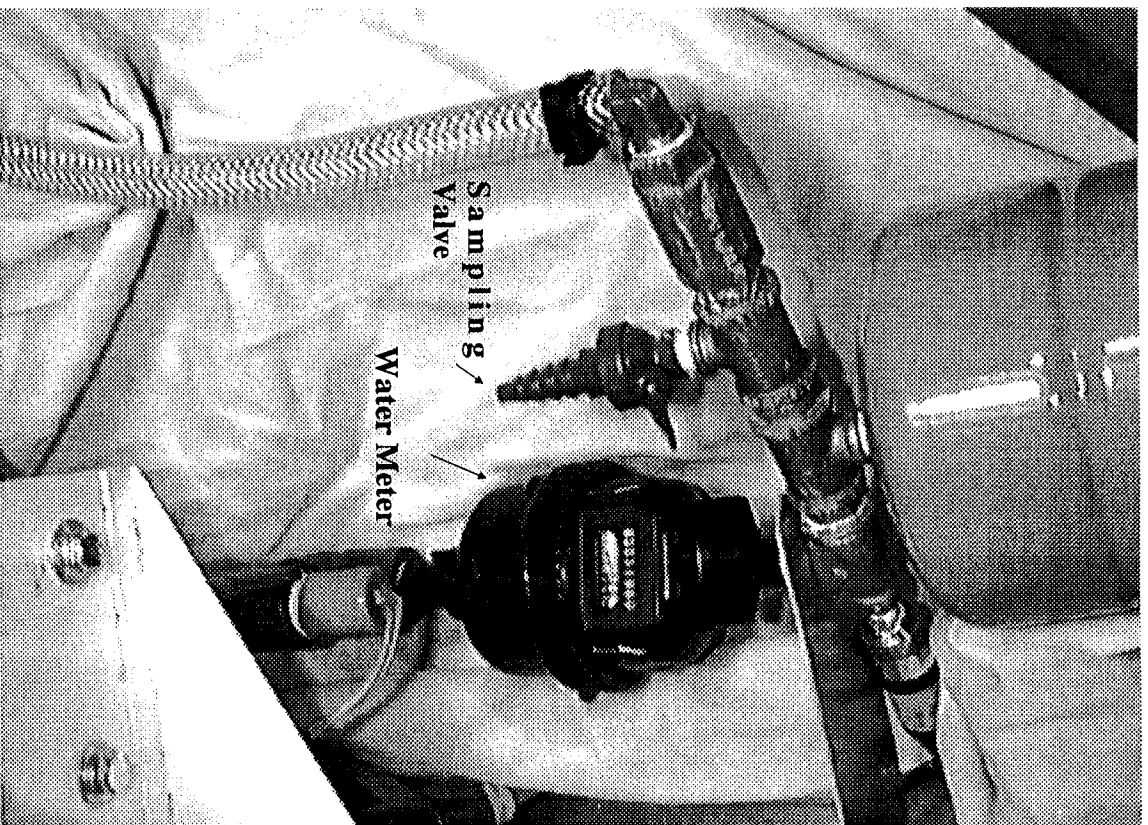
Dia. 5 Water Meter and Carbon Filter Sampling Valve
